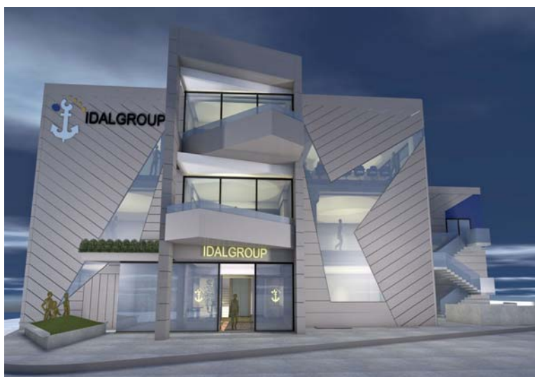
Idal Group scarl – Energy Building Salerno (SA)
